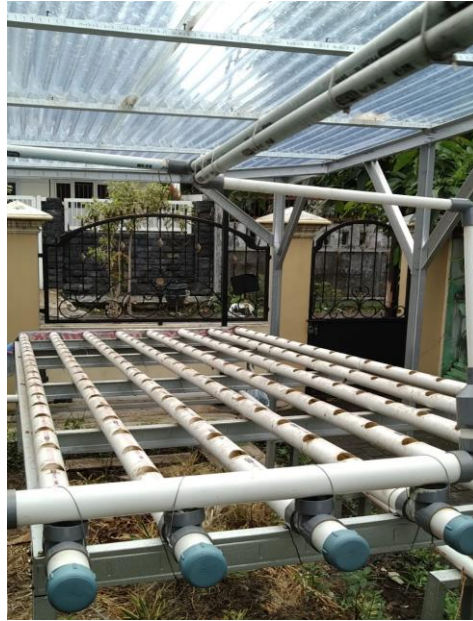
Figure 8. Hydroponic Plant Pipe
