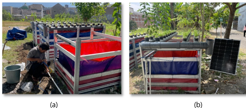
Figure 2. Aquaponics making activities applied in Sunan Kalijaga Mosque: (a) Making aquaponics framework, (b) Installing solar electricity
