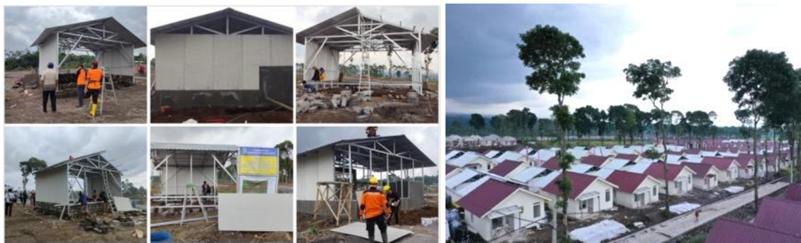
Figure 2. a) Temporary housing structures and materials. b) New settlement
