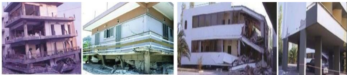
Figure 3. Examples of the impact of earthquakes on buildings [4]
