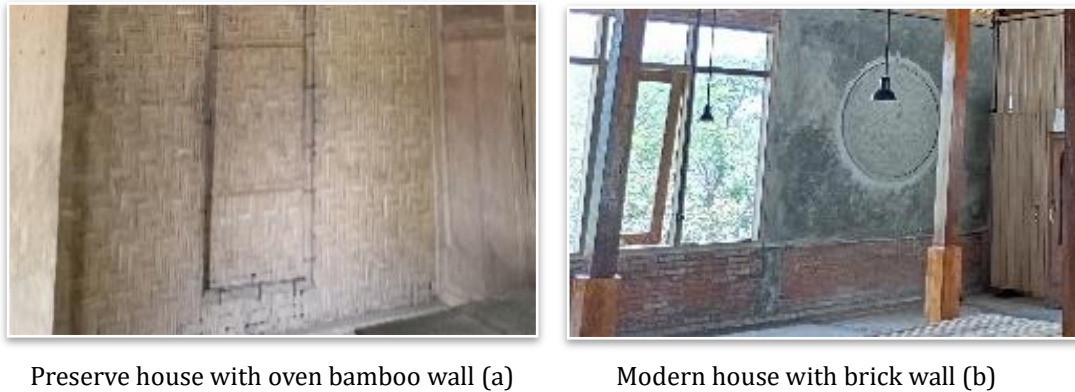
Figure 8. Comparison of wall materials between traditional and modern Limasan houses.
