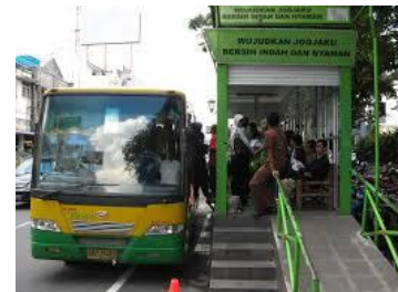
Figure 21. Bus stop for BRT Passengers
