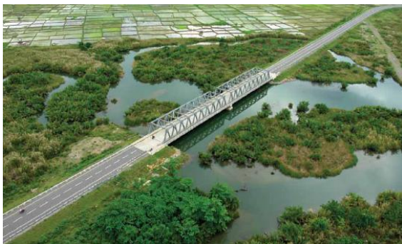
Figure 4. Green infrastructure area in rural road (Source: Purdue Land Use Team, 2007)
