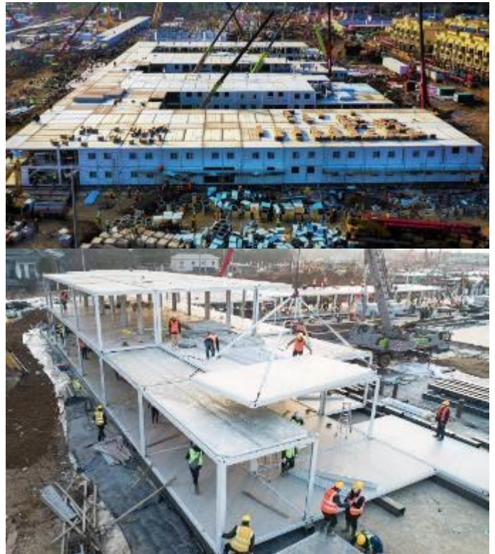
Fig. 5. Honshenshan Hospital Distrik Caidian Wuhan Cina [10]
